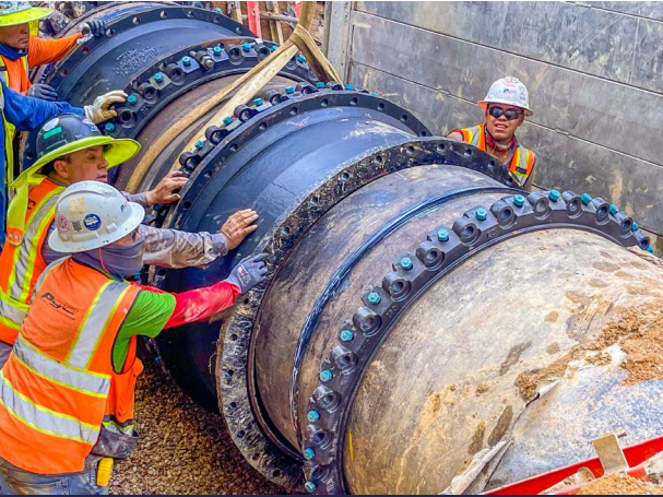
SOUTHWEST AUSTIN 48-INCH LINE REPAIR | JUNE 2024
