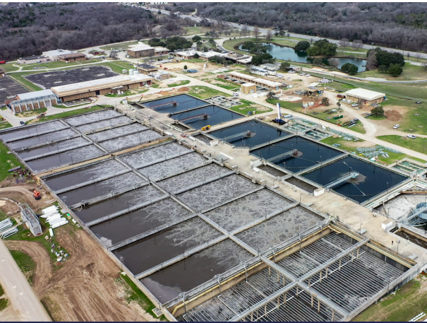
WALNUT CREEK WASTEWATER TREATMENT PLANT
